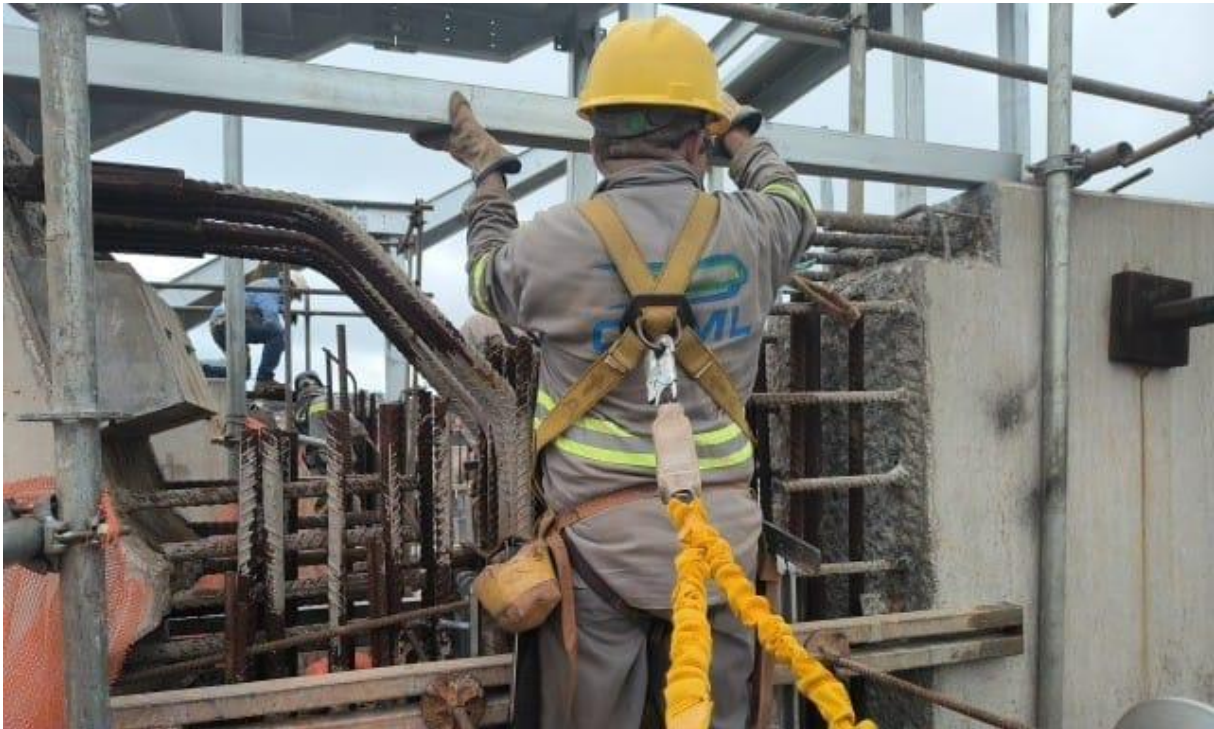
Figure 21: Preparation to install the base plates (Source: São Paulo Metro, 2026)
