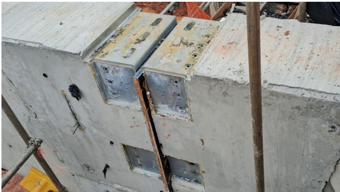
Figure 24: Removal of the blind plates after concrete placement (Source: São Paulo Metro, 2026)
