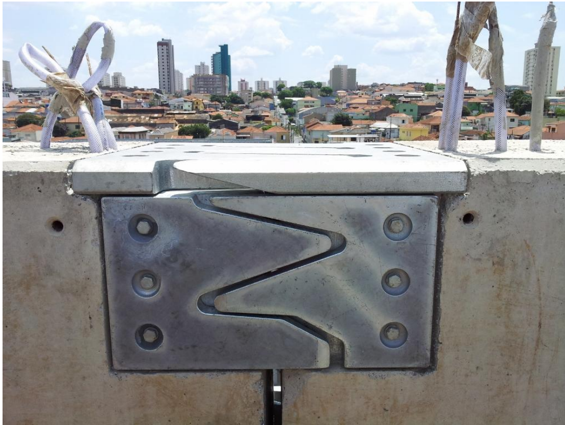
Figure 25: Finger plates installed following bolt installation per procedure
