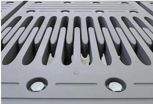
Figure 7: Samples of textured finger plates (Source: Maurer SE)
