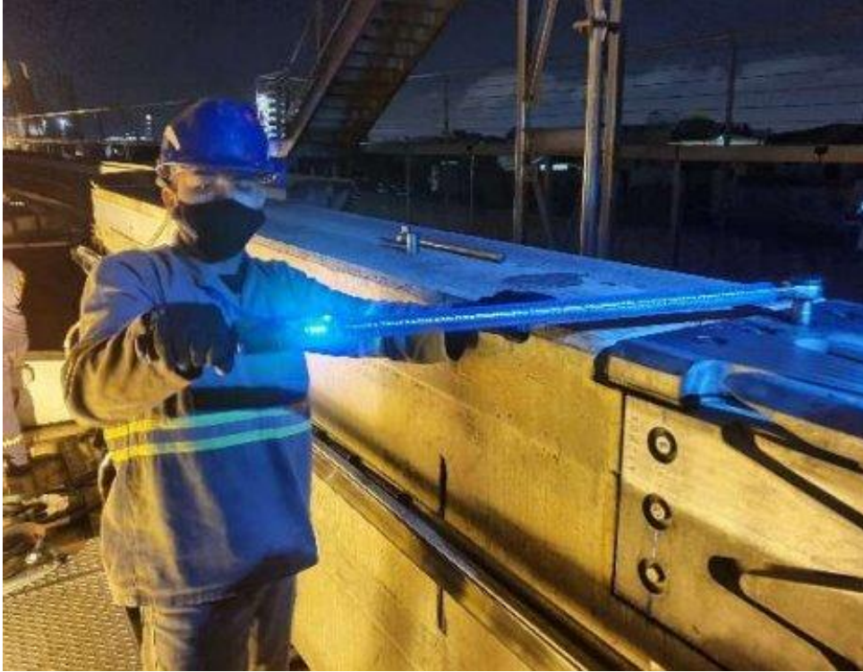
Figure 26: Sample of a torque angle method application
