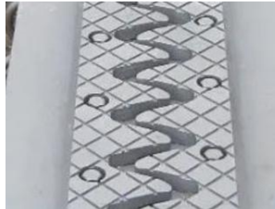
Figure 7: Samples of textured finger plates (Source: Maurer SE)
