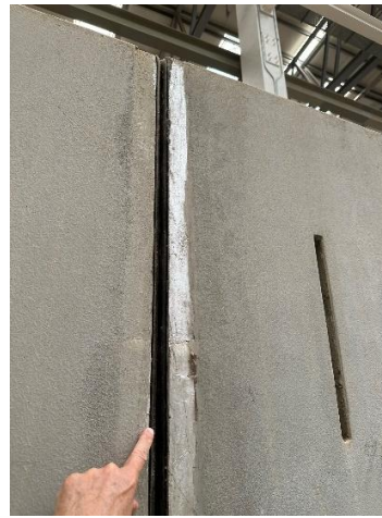
Alstom — Depot, East of Nile Line, Cairo
