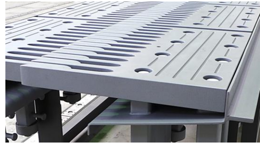
German Highway authority, A45, Wetzlar
