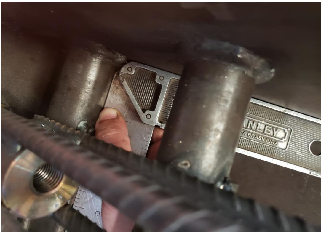
Figure 17: Verification of the anchor orthogonality (Source: Rodolfo Szmidke, 2021)
