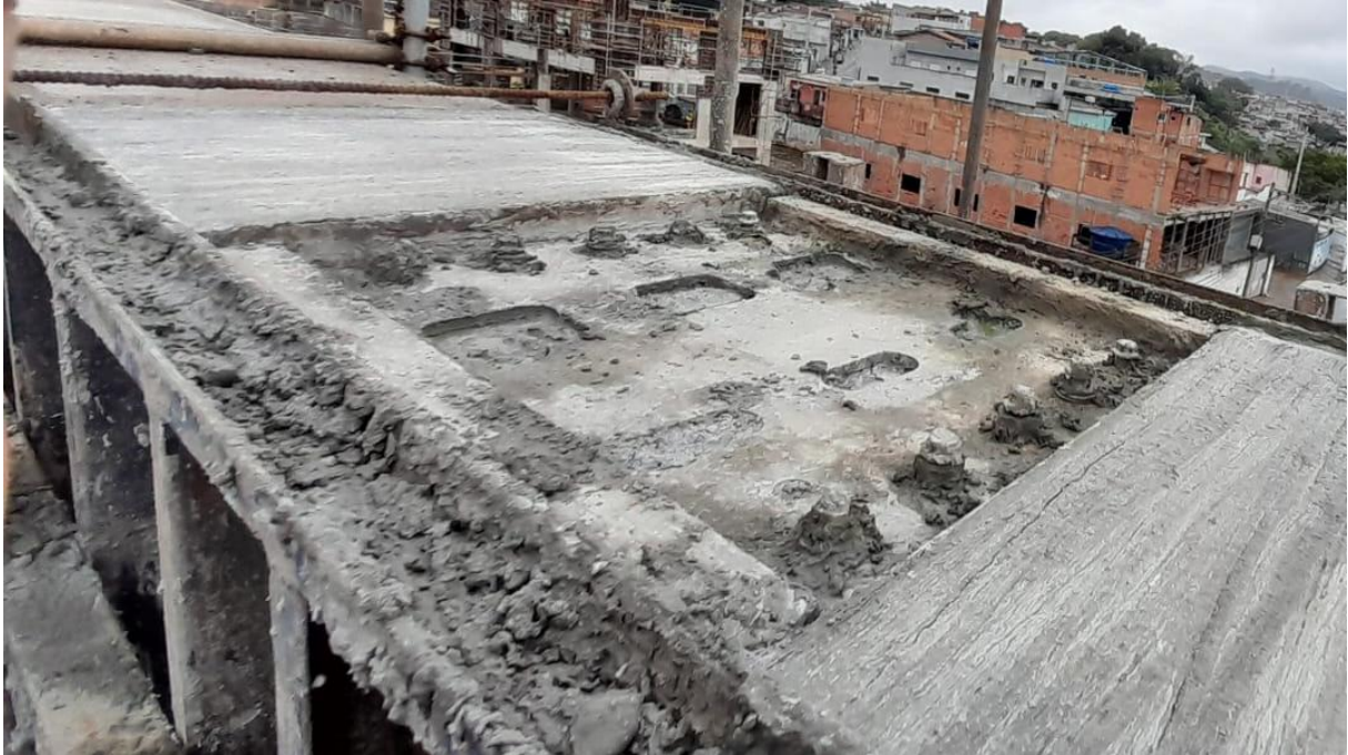
Figure 23: Note the concrete filling the holes in the base and blind plates (Source: São Paulo Metro, 2026)
