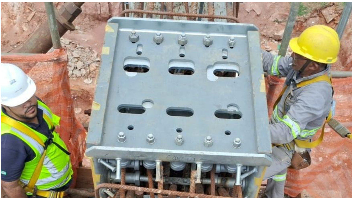
Figure 22: Installation of the blind plates (Source: São Paulo Metro, 2026)
