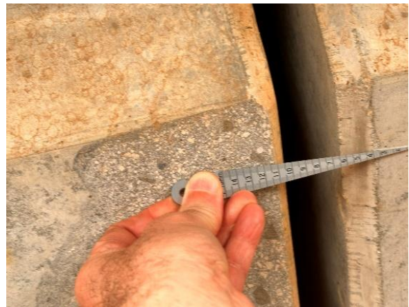
Hitachi — Depot, Panama Line 3 (expansion joint detail)
