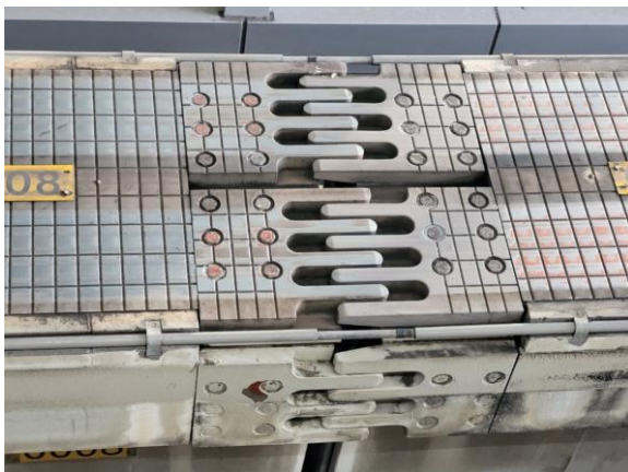
Figure 8: Samples of textured monorail finger plates from Kitakyushu Monorail (Source: Rodolfo Szmidke, 2024)
